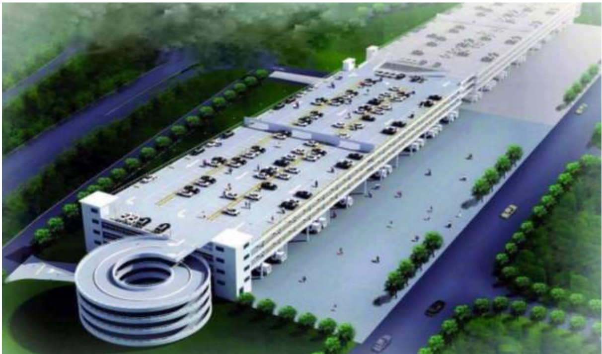
Figure 2: (Multi-storey car park project)
