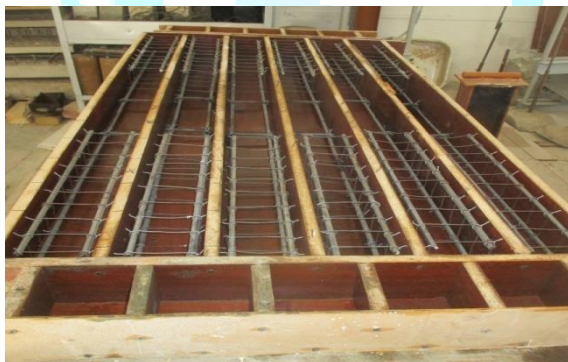
Fig.3. Crossbar formwork
