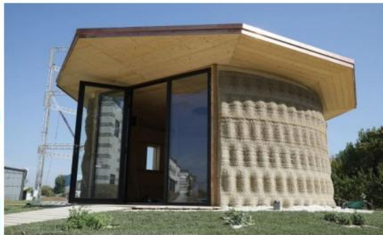
Figure 6 - Gaia Residential Building
