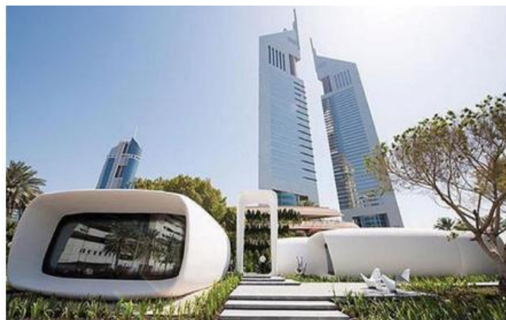
Figure 2 - Office complex in Dubai
