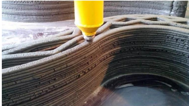
Figure 1. Layer-by-layer application of the mixture using a 3D printer
