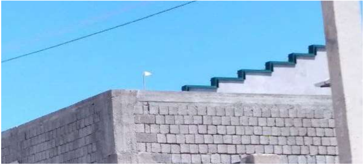
Pictures 2 and 3. Incorrect retransmission system in the antenna installed and used by the entrepreneur.
