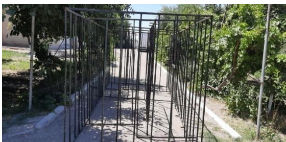
4-picture. Maze-shaped two-way movement barrier.
