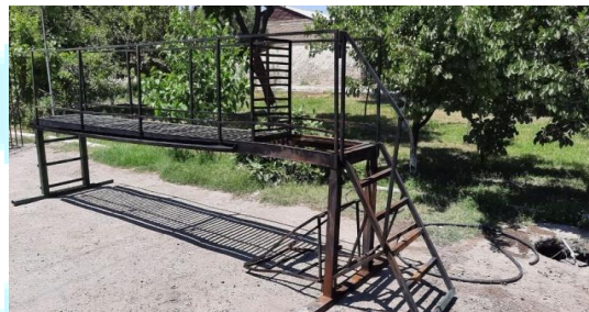
6-picture. A grid bridge mounted on a concrete pool to pass through the flames.
